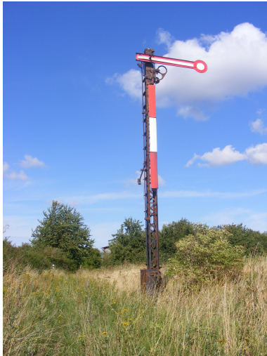
(Ger.) Signalmast, Formsignal
